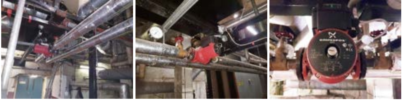
The single head circulation pump for the heating coil on teaching pool air handling unit
