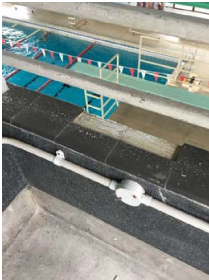
Fig 4.4.7 – The photo above was taken within the main pool area on the second-floor galleries showing a close-up view on the existing broken / missing tiles on the gallery parapets.
