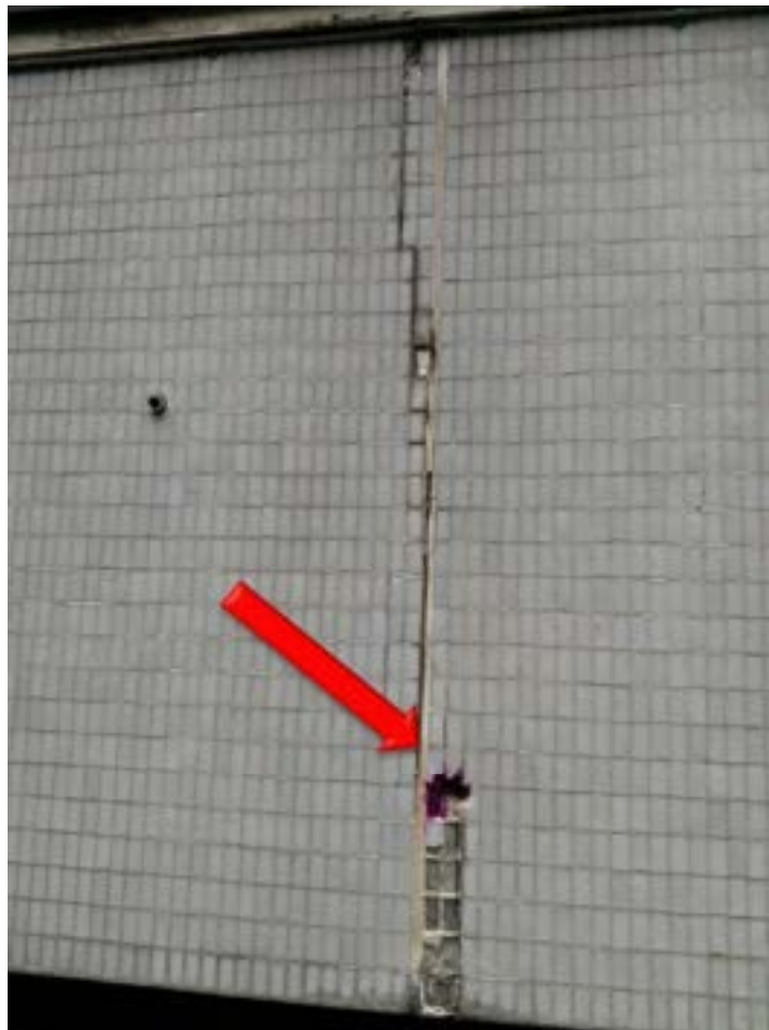
Fig 5.1 – The photo above shows a typical example of potential tile shelling at movement joint in the facade.
