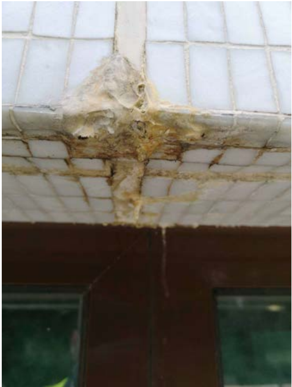
Fig 5.2 – The photo above shows a typical example of potential tile shelling at movement joint in the façade and an historic repair.
