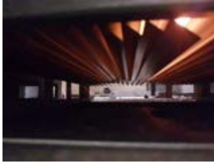
The clean burner frontage on boiler 5 and an evenly burning flame.
