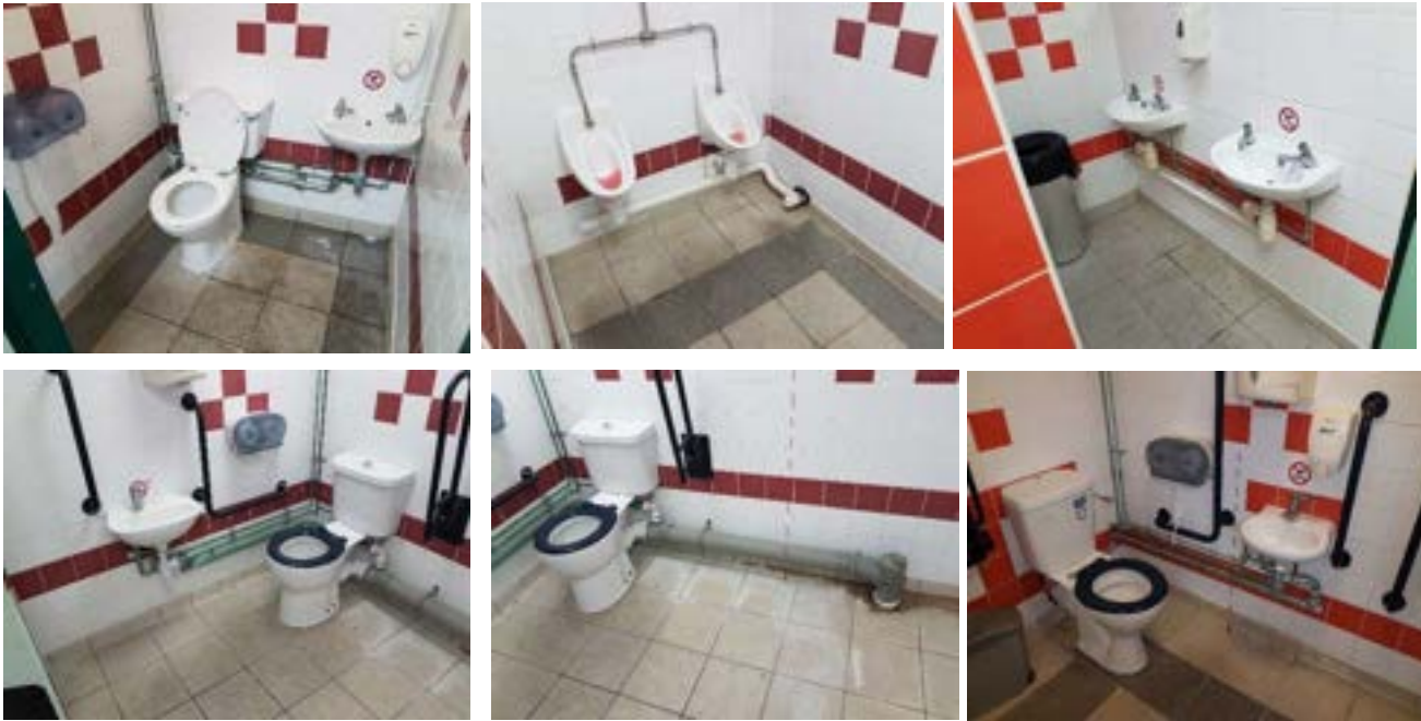
A selection of wc pans and wash hand basins drain connections showing a few leaks and generally tired.
