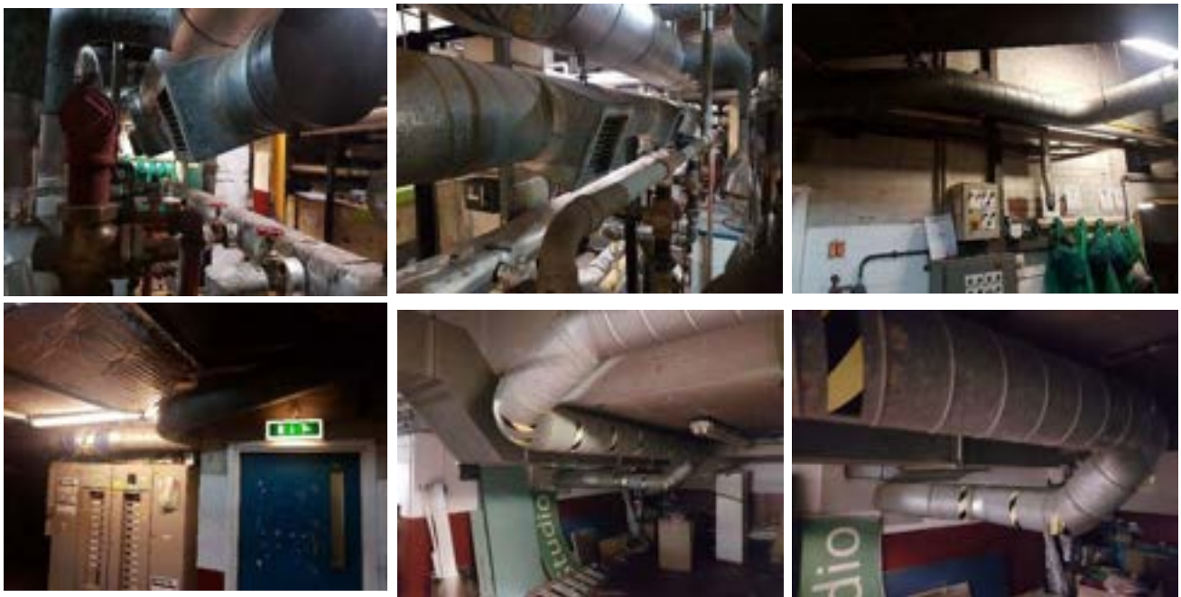
The boiler combustion air extract system showing the 3 no. grilles above the boilers, the ductwork at high level, the cased axial extract fan located above the main electrical distribution for the building and where the system enters the old fresh air plenum.
